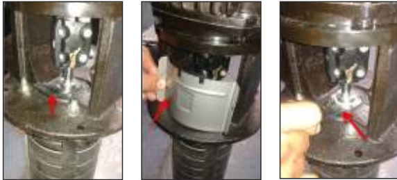
fig 10 Procedure of float gauge removal
